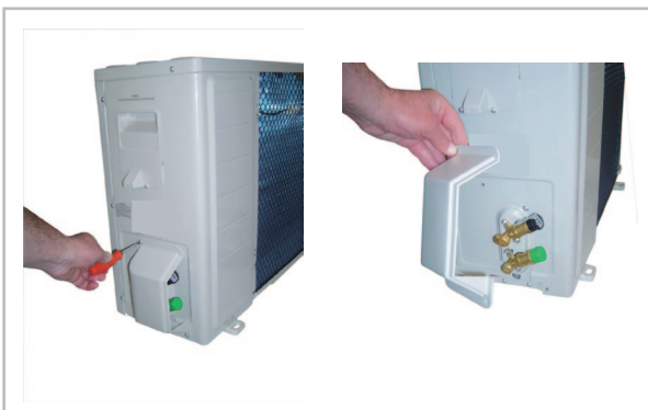
Fig. 19: Remove the plastic cover
