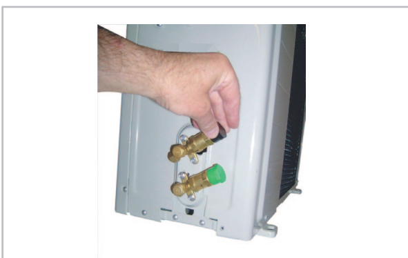
Fig. 20: Remove protective caps
